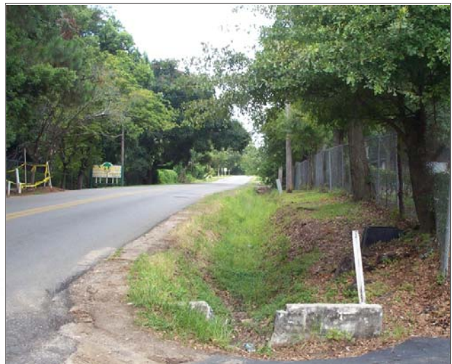
Open drainage ditches along neighborhood streets are a hazard to pedestrians and drivers alike
